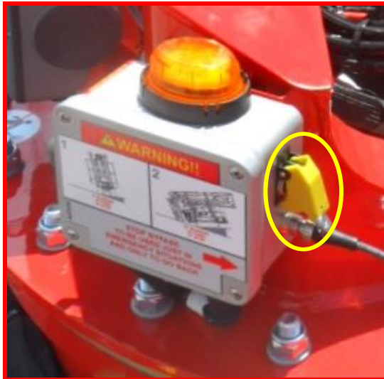
Picture 24: electric box for travel block bypass.
